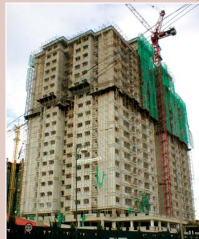
Dataran Prima Condominium Phase 1 (under construction)
