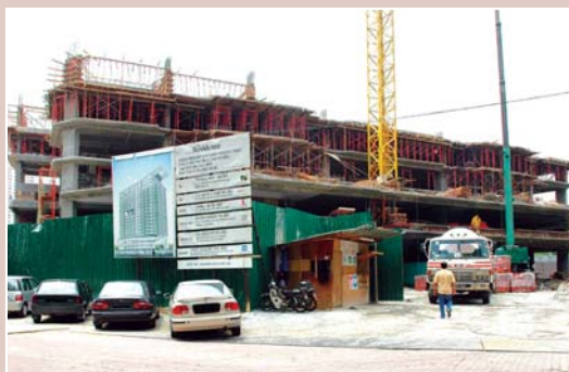
Residence Condominium, Taman Tun Dr. Ismail (under construction)
