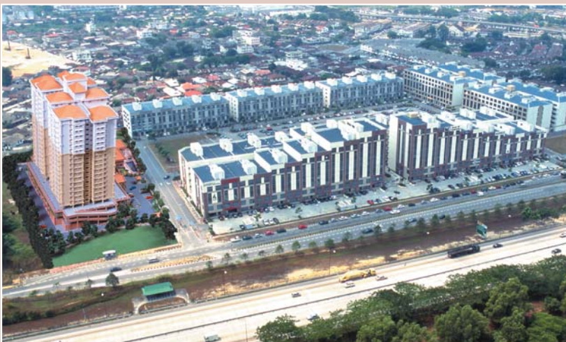
Dataran Prima Commercial Centre & Condominium
