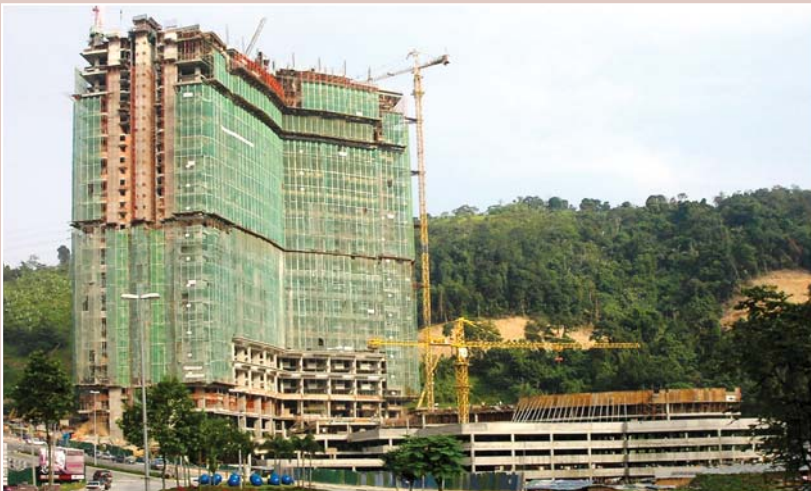
Armanee Terrace, Damansara Perdana (under construction)
