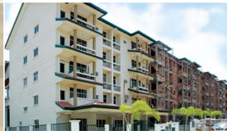
Taman Lagenda Mas 2B - Townhouse, Cheras, Selangor. (under construction)
