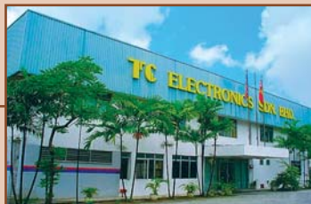
T.C. Electronics Factory, Port Klang.
